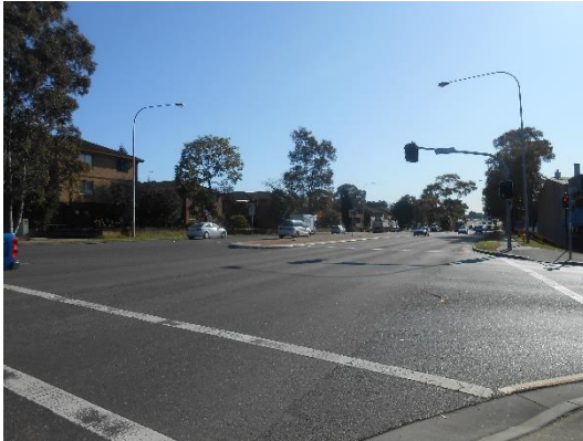
Figure 2.2: St Hilliers Road (looking North)
