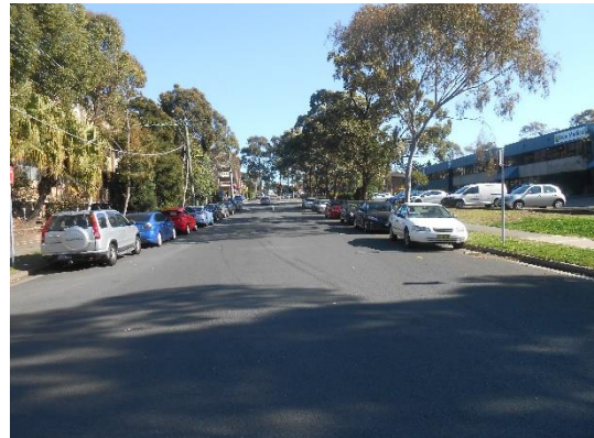
Figure 2.5: Hall Street (looking West)
